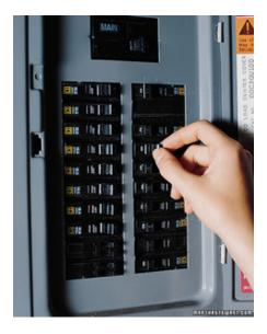
operating an appliance with too high a voltage or wattage requirement for the circuit. The sudden starting of an electric motor can also trip a breaker. If a breaker trips repeatedly check for any of the above causes.
